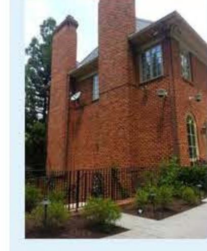
Photo courtesy of Home Fronts News Right side elevation to a house in McLean soon to be augmented by a four-stop elevator.
