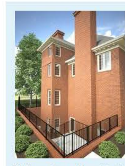
Photo courtesy of Home Fronts News A McLean couple in their late-60s had Glickman design a 60-foot 4-level elevator tower on the home's right elevation. The tower will be re-clad in brick that matches the existing masonry and will not be visible from the front facade.
