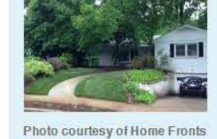
Photo courtesy of Home Fronts News When Jaime Marquez began having difficulties getting from the house to the driveway, Glickman Design Build created a graduated front walk for the Arlington family. The new walk rises one inch per foot. The plan included replacing a front stoop with a "zero step" entry and widening interior doors and halls.
